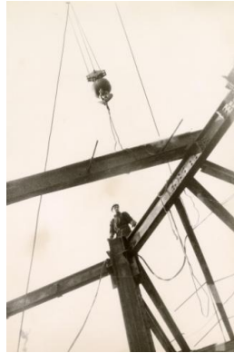
Title: Construction worker supervising iron beam placement while standing on high beams
