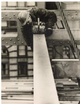
Title: Construction worker fixing beam with tool box Date: c. 1955 Primary Maker: Jacques Lowe Medium: Vintage gelatin silver print
