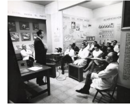
Title: Builders and doctors in Brasilia: Brasilia, the most modern capital city in the world has 65,000 inhabitants in 1959. Today, its population totals 250,000. In three years, this figure will increase to 500,000. Since the first foundations were laid, builders and doctors have worked closely together, first to see to it that the 60,000 workers who took part in building the new city stayed in good health; then to prevent the town from being invaded by diseases of the bush and forest. Immigrants' health are checked systematically on the roads in order to discover possible sources of dangerous disease. Date: c. 1960 Primary Maker: Paul Almasy Medium: Vintage gelatin silver print
