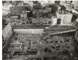
Title: Construction site on West 52nd Street Date: c. 1955 Primary Maker: Jacques Lowe Medium: Vintage gelatin silver print
