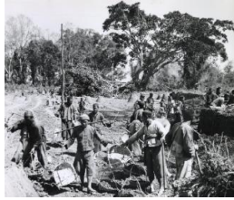
Title: Building the railbed of the Yunnan, Burma
