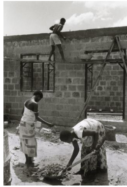
Title: Women digging hole help to construct house, Ghana
