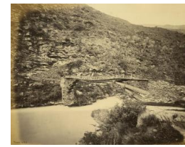
Title: Bridge Across the Sutlej on the Kulu Road Date: c. 1866 Primary Maker: Samuel Bourne Medium: Albumen print
